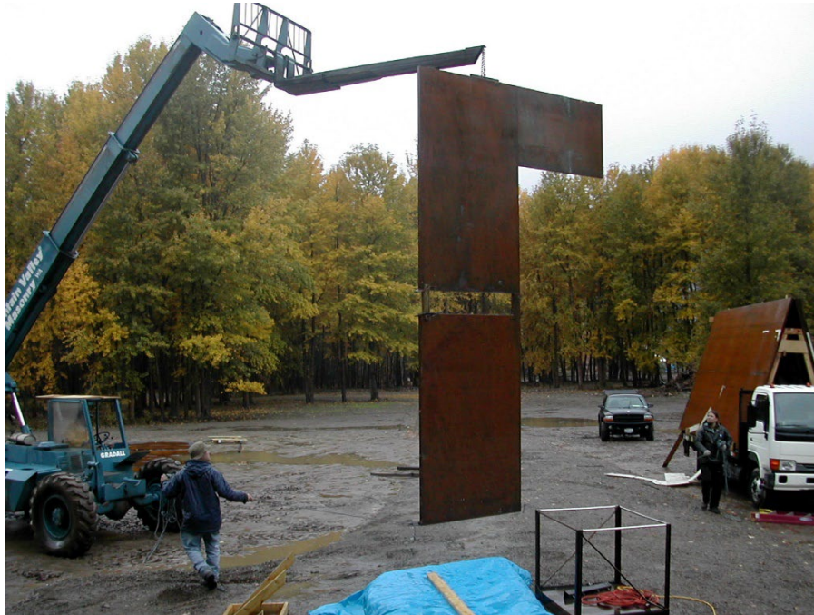
Figure Q1d: Delta shelter exterior cladding.
